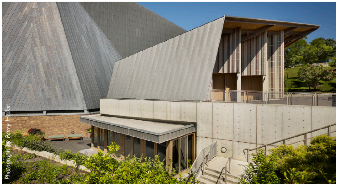
The two-story pavilion activates the main plaza by serving concessions and at the lower level teaches students at the education center and engages donors on the private plaza.
